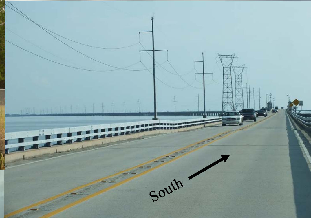
Goose Point Fault offsets Hwy 11 Bridge
